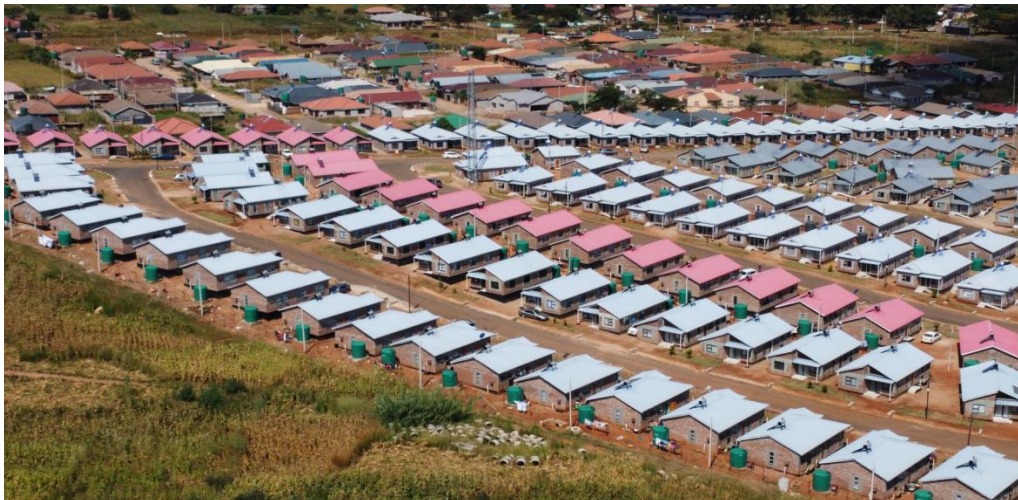
Kuwadzana FBC Housing Project
