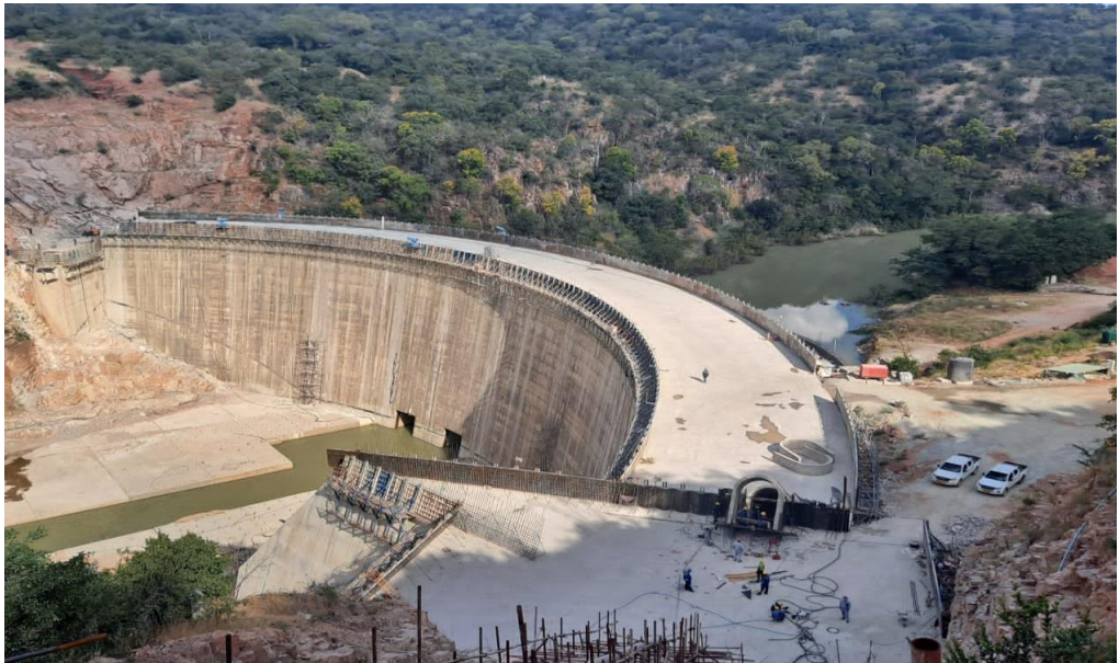
Gwayi Shangani dam
